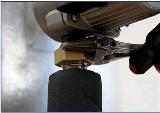
12. Insure the pump connection is tight.
