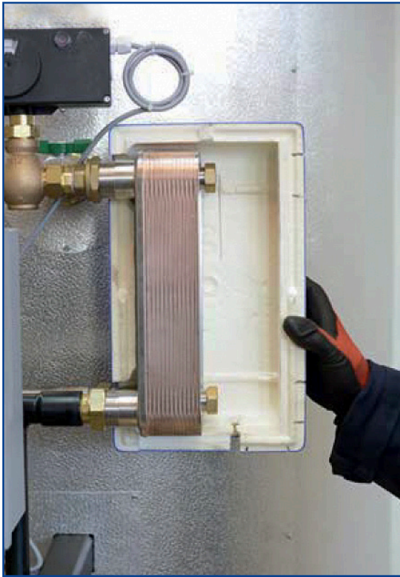
15. Mount the first half of the insulation jacket, aligning with the heat exchanger secondary connections.
