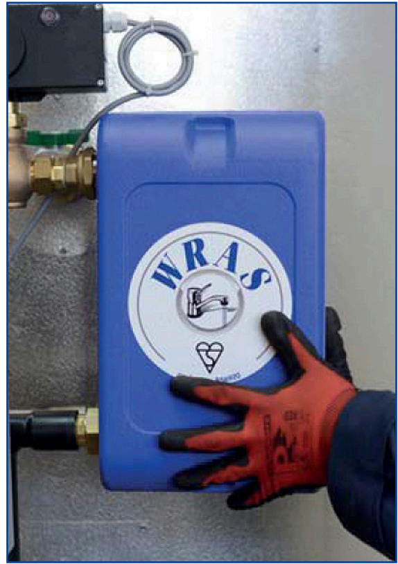
16. Mount the second half of the insulation jacket, aligning with the heat exchanger primary connections.
