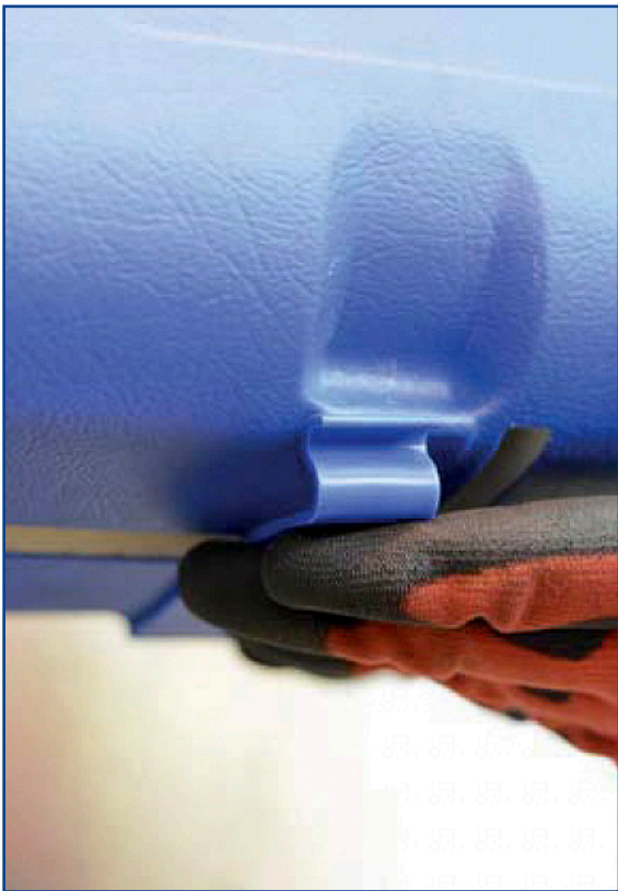
17. "Snap" on the insulation retaining clips.
