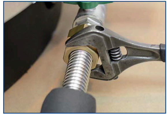
13. Install a fibre washer in the flexible hose and connect to the bottom connection on the AquaSTOR.
