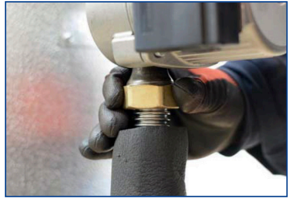
11. Connect the flexible hose to the secondary pump.
