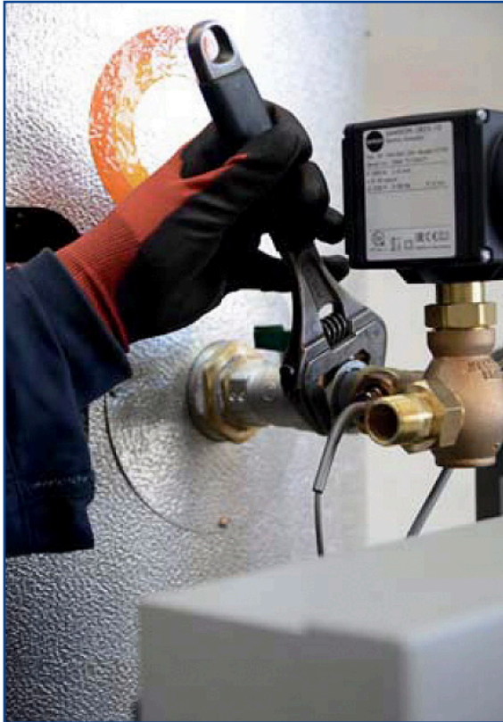
5. Mount the heat exchanger on the support bracket and connect to the secondary isolation valve.
